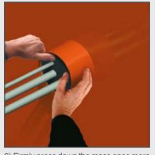
9) Firmly press down the mass once more by hand. This is extremely important to ensure effective conductivity. Then apply the CONDUCTON® flexible rubber at the other side of the penetration in a similar way.
