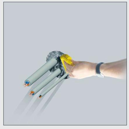
9) The FIWA® sealant between the cables is pressed down and smoothed by hand or with a spatula or putty knife.
