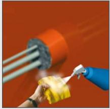
11) To smooth the surface of the FIWA® sealant layer, a cloth is sprayed with water.
