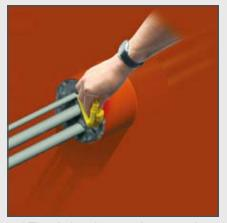
12) The cloth is then used to press down the sealant layer. People with sensitive skin should use gloves when working with the FIWA®.
