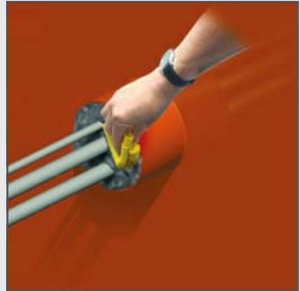
12) The cloth is then used to press down the sealant layer. People with sensitive skin should use gloves when working with the FIWA®.
