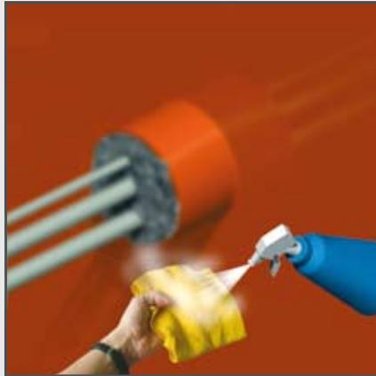
11) To smooth the surface of the FIWA® sealant layer, a cloth is sprayed with water. This prevents the sealant from sticking to the cloth.
