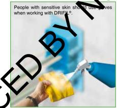
14) To smooth the surface of the DRIFIL<sup>®</sup> sealant layer, a cloth is sprayed with water. This prevents the sealant from sticking to the cloth. Note: do not use soap water!
