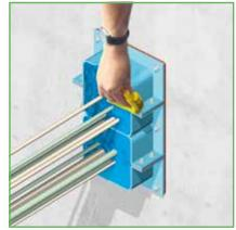
15) The cloth is then used to press down the sealant layer. People with sensitive skin should use gloves when working with DRI-FIL<sup>®</sup>. Please refer to the Safety Data Sheet for more information.
