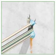
1) Occasionally it is impossible to remove an existing seal in an opening. In this case, just remove the protruding portion of the seal and utilize a CSD<sup>®</sup> split flanged frame and the RISWAT<sup>®</sup> system.
