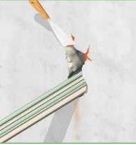
2) If there are large irregularities in the wall around the opening, they should be locally smoothed with DRIFIL<sup>®</sup> or NOFIRNO<sup>®</sup> sealant. NOFIRNO<sup>®</sup> sealant has highest mechanical properties.
